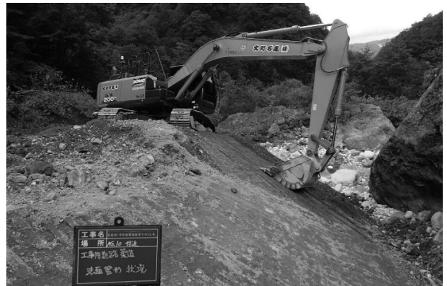
図-9 ICT法面整形
