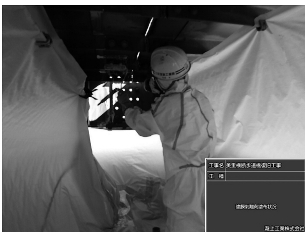
図-6 塗膜はく離剤塗布状況
