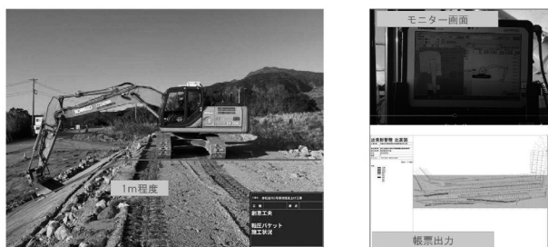
図-6 施工端部・法面の締固め (ICT)
