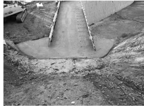
図-6 左岸側間詰
