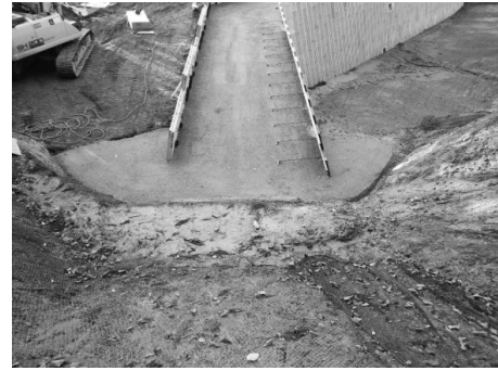
図-6 左岸側間詰
