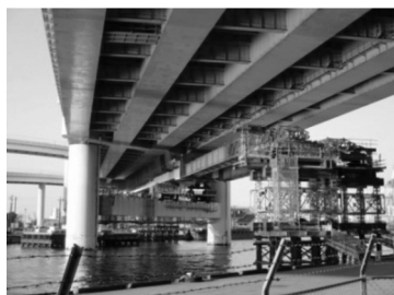
図-6 送り出し架設状況
