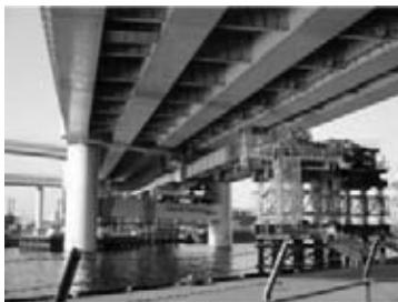
図-6 送り出し架設状況
