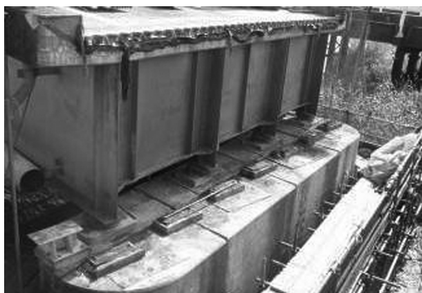
図-9 桁扛上前 (P3 橋脚)
