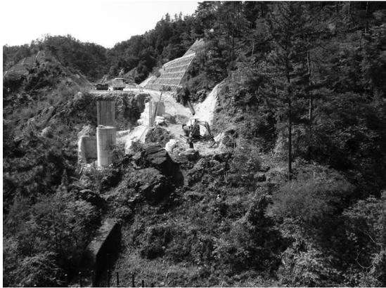
図-3 桁干渉部岩山掘削況
