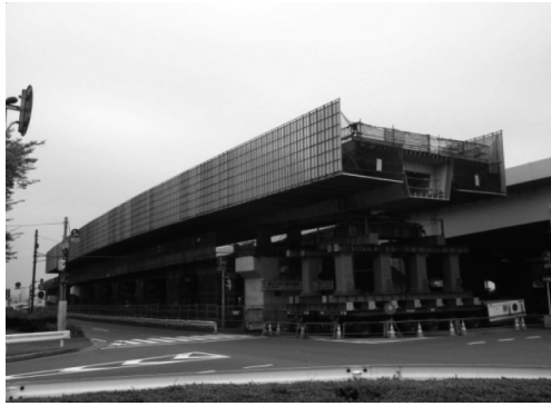
(a) 送り出し架設前
