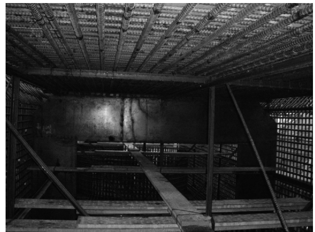
図-6 誘発目地設置状況
