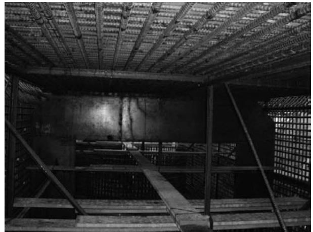
図-6 誘発目地板設置状況
