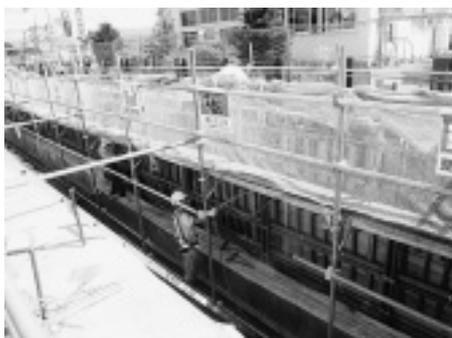
写真-4 打設時型枠散水冷却
