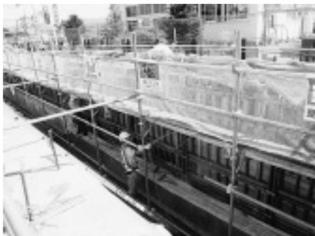
写真-4 打設時型枠散水冷却
